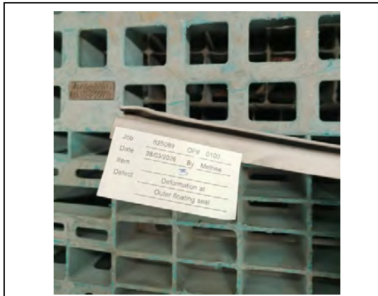
Fig.25 Deformation on outer floating seal.
