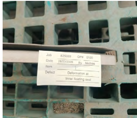
Fig.20 Deformation on inner floating seal.
