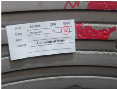
Fig.15 Heavy corrosion across body.
